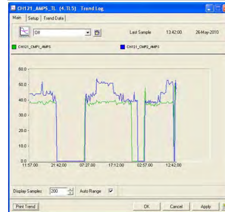
CHILLER TREND LOG
